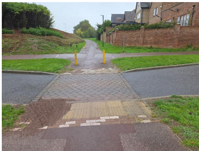
Damaged and incorrectly reinstated Give Way markings.
